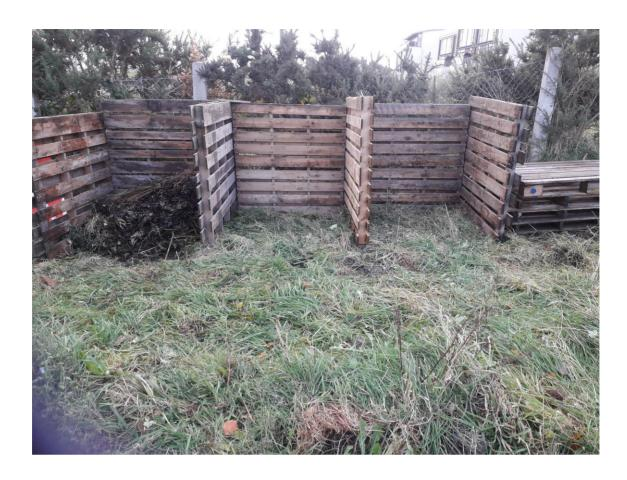
CTT recently constructed a composting system to make our practices more sustainable. All those leaves and organic waste will soon be converted into compost for 2020. The fresh stuff goes in on the left-hand side and after forking into adjacent bins, the home-made compost should come out on the right-hand side. It was a cold day for this job! Many thanks to The Foy Centre for letting us use this spot at the corner of the football field.
